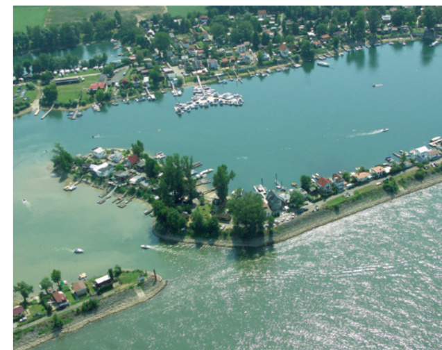
Flooded every few years: The sewer system installed by Roediger® is leak-proof even under the most extreme conditions.
